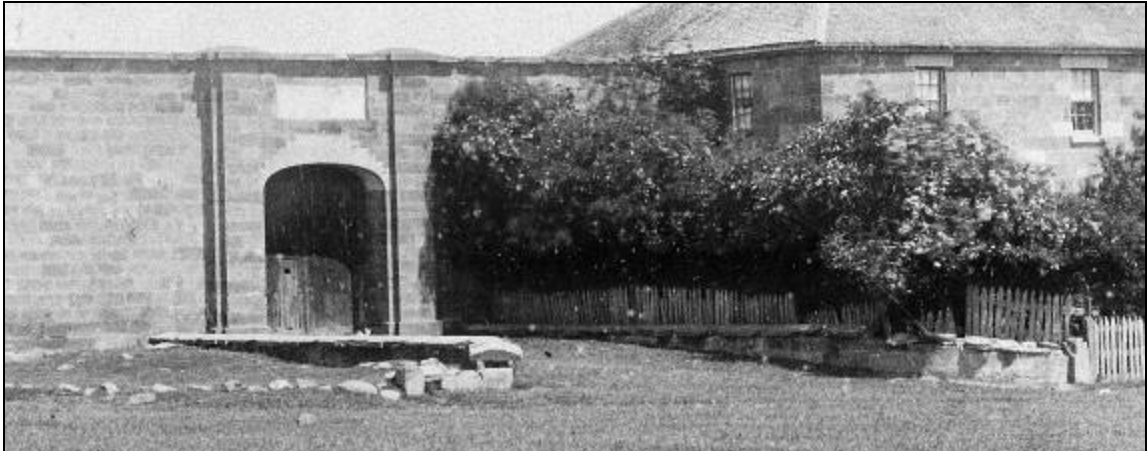
Plate 13.2 – The gaol arch and gates c1910. This photograph clearly shows the approach wingwalls and raised platform (bottom-left) where the gallows may once have stood. Photograph – Allport Library, State Library of Tasmania.
