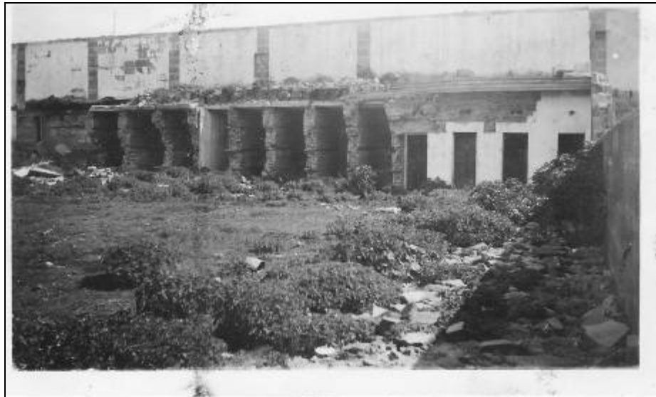
Plates 7.3 & 7.4 –Demolition of the Men's Division, late 1937. Photographs courtesy of Graeme Raphael, Oatlands (top) and the Oatlands District Historical Society (bottom).
