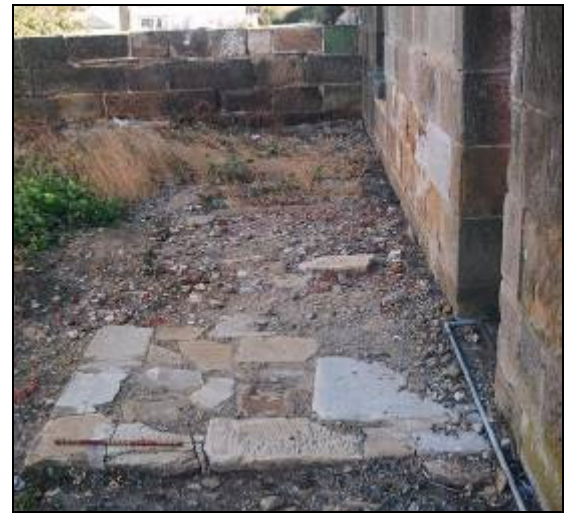
Plate 13.9 – Foundations of a skillion at the back door of the Gaoler's residence.
