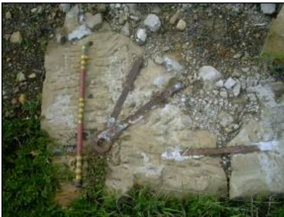
Plate 13.4 – Foundation of western main gate pillar showing iron cramping and hinge support.
