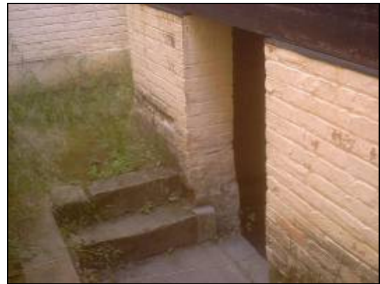
Plate 13.17 – Steps leading to the semi-basement of the Hobart gallows
