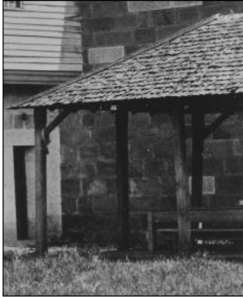
Plate 13.19 – Part of the open timber shed in the Debtor's Yard. Photograph – State Library of Tasmania.
