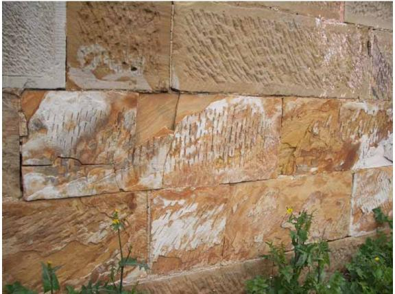
Figure 7 – Efflorescence of salt on the face of stone. Whilst the exfoliation is probably a result of face bedding, continued salt attack will accelerate this (note also pointing loss).
