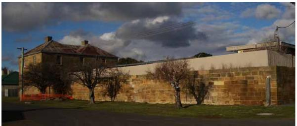
Figure 5 – The western wall of the gaol (the Gaoler's residence at left). The perimeter wall shows signs of damp (dark patches) and efflorescence of salt (white patches) even at this distance.
