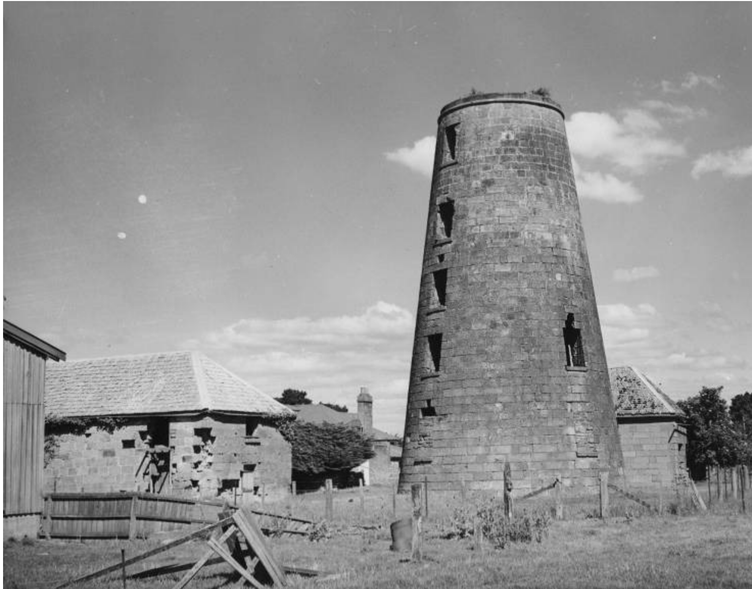
Figure 2.24 – Callington Mill in 1966, taken by Sir Ralph Wishaw. TAHO NS165-1-333
