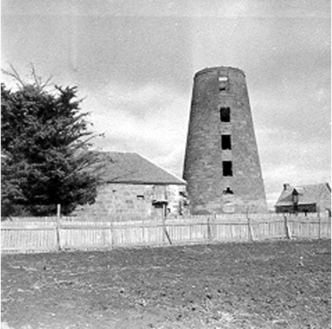
Figure 2.22 – Callington Mill late 1940s showing the rear of the granary, note that the ruins of the steam mill had been demolished (TAHO PH30/1/4917).
