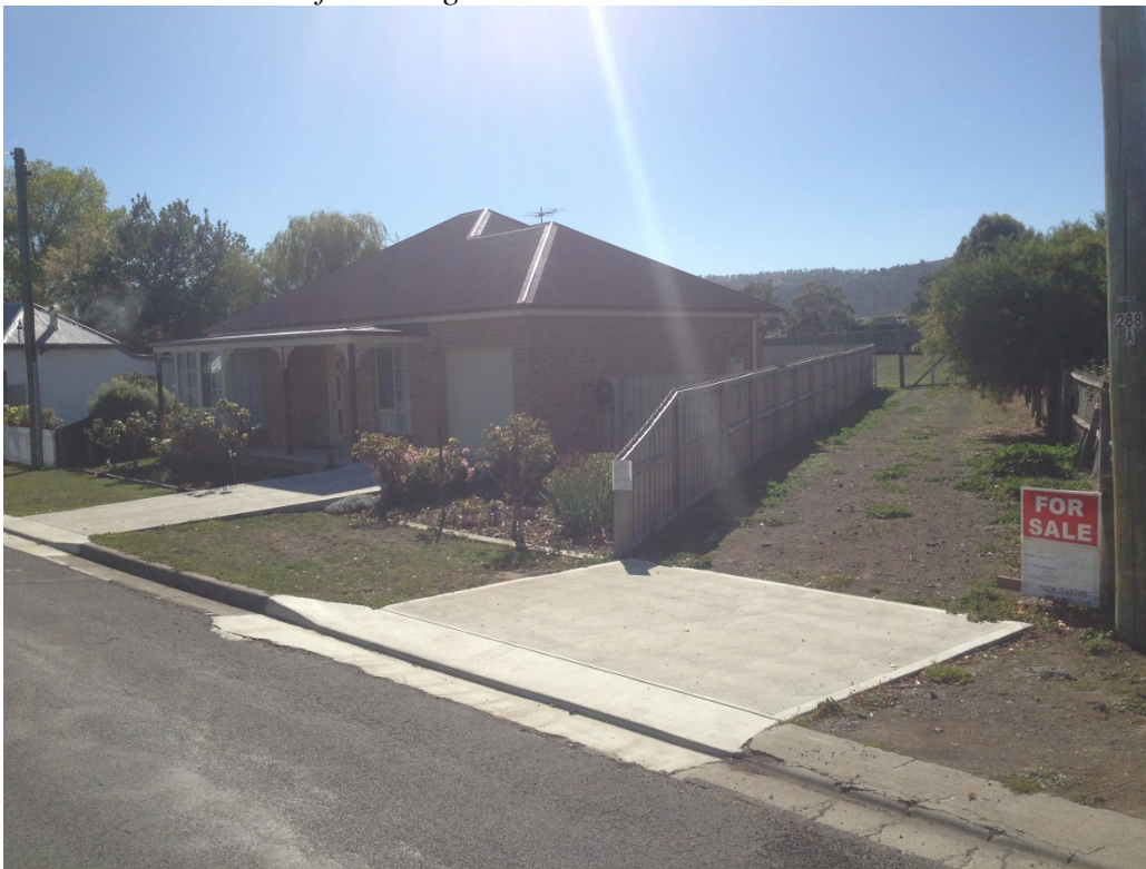
Photo 2 – The red roof dwelling is 72 Main Street. The concrete access, in the foreground, is the access to 70A Main Street.
