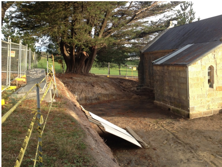
Rear cut area – Mid 2014
