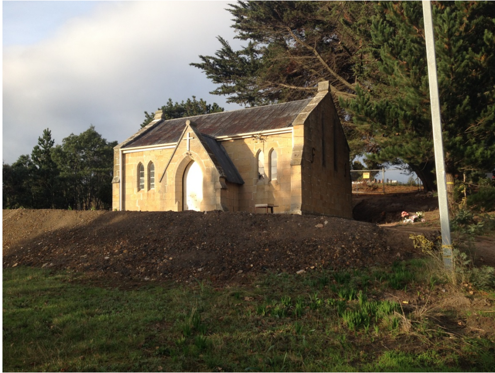
Front view of the church showing the fill embankment – Mid 2014
