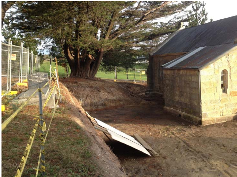
Rear cut area, showing proximity of nearest grave.
