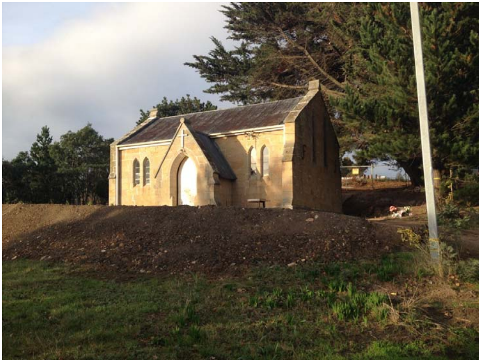
Front view of the church showing the fill embankment
