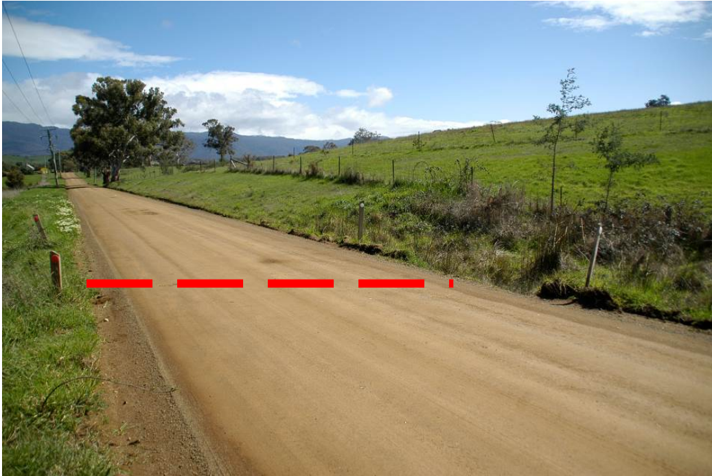
Photo 4_ This culvert would need to be widened to achieve a 6m pavement width with shoulders. The dashed red line marks the approximate position of the culvert. Photo was taken looking west
