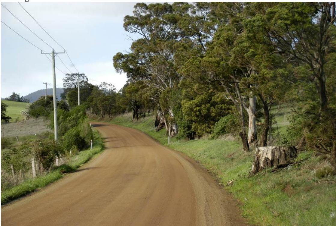
Photo 3_ More possible tree removal and embanking may be necessary along this part of the road to achieve a minimum 6m width with shoulders. Photo was taken looking east.
