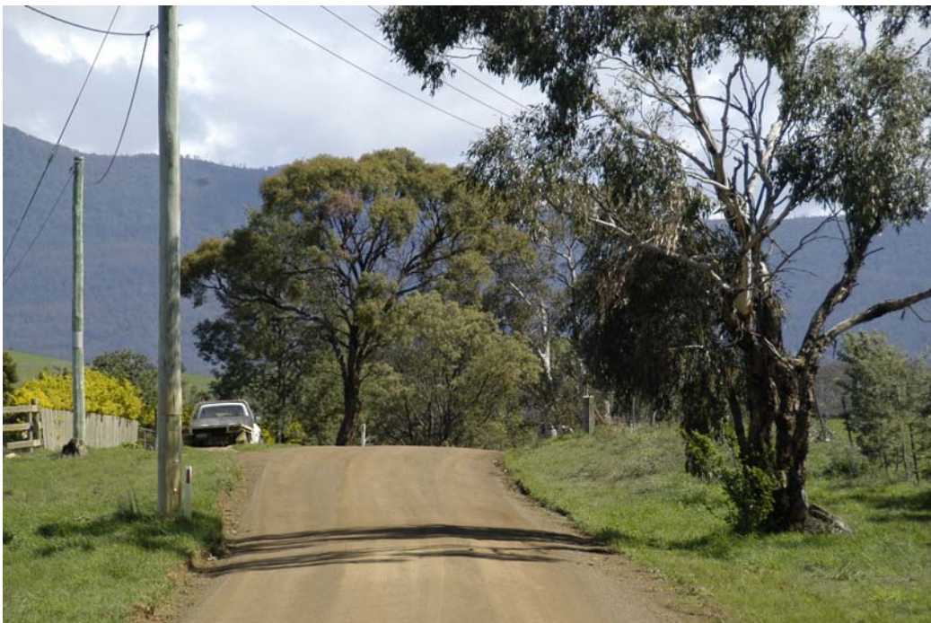
Photo 5_ the left hand side of this photo is the house nearest to the road along the cartage route. Some reshaping of the corner and widening would be necessary in this section. Photo was taken looking west.
