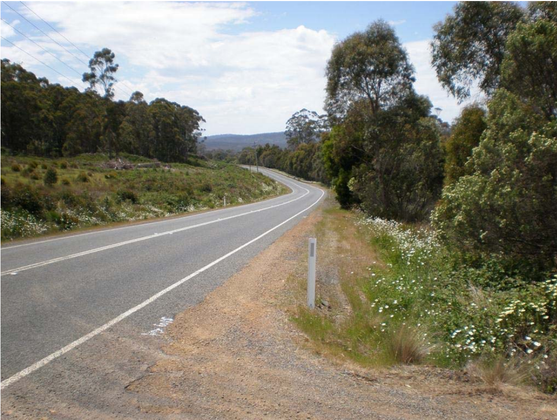
Site Distance to Lot 3 quite Good. Proposed Lot 1 Access is located approx 50m south of this access.
