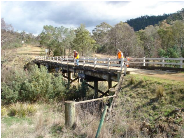
Existing Swanston Bridge
