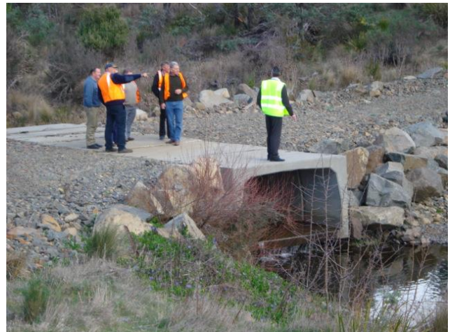
Existing Swanston Bridge Bypass
