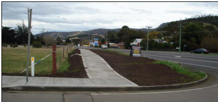
East Bagdad Road / Midland Highway footpath
