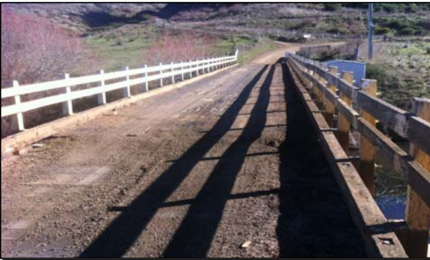
The old Rotherwood Road bridge deck structure
