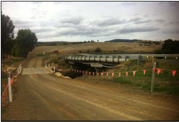
The old Brown Mountain Road Bridge (showing the bypass)
