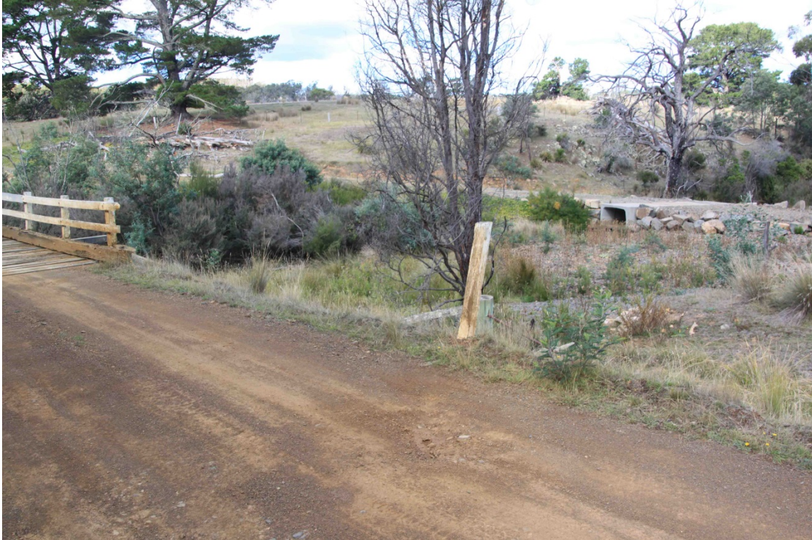
Heavy vehicle bypass culvert from the west abutment of the Swanston Bridge.
