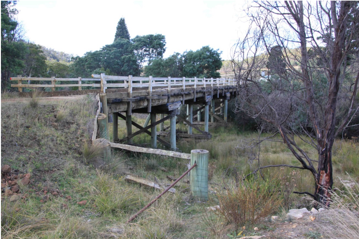
Swanston Road Bridge over the Little Swanport River from south-west abutment
