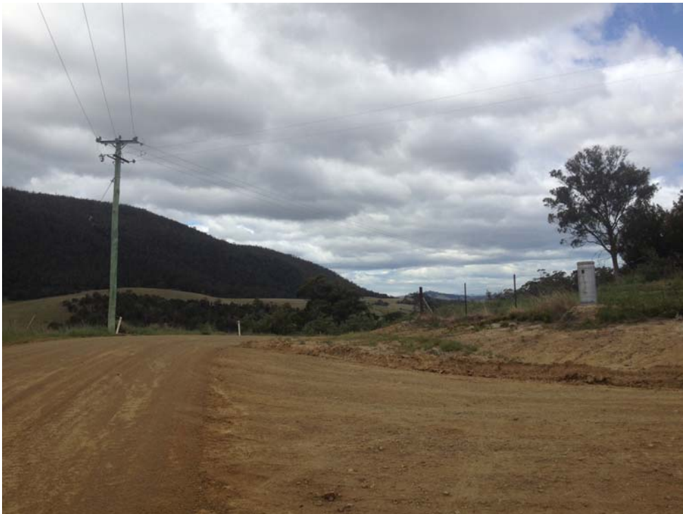
Photo 3_ sight distance to the south east at only 40m. Sight lines are obstructed by the embankment on the corner of the road.
