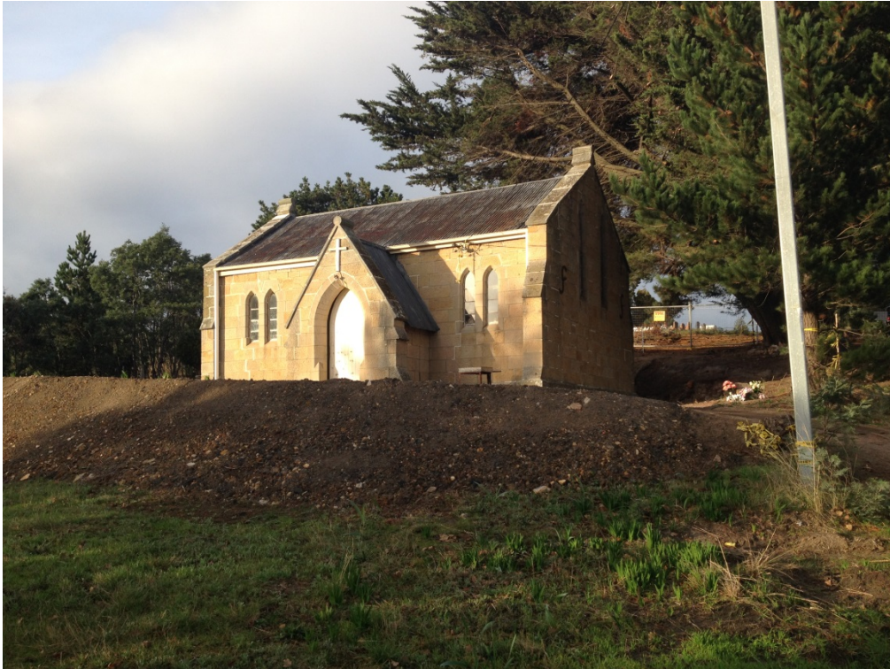
Photo 4_Photo demonstrates the fill and a possible car parking space on the 'Church Lane' side of St Anne's.
