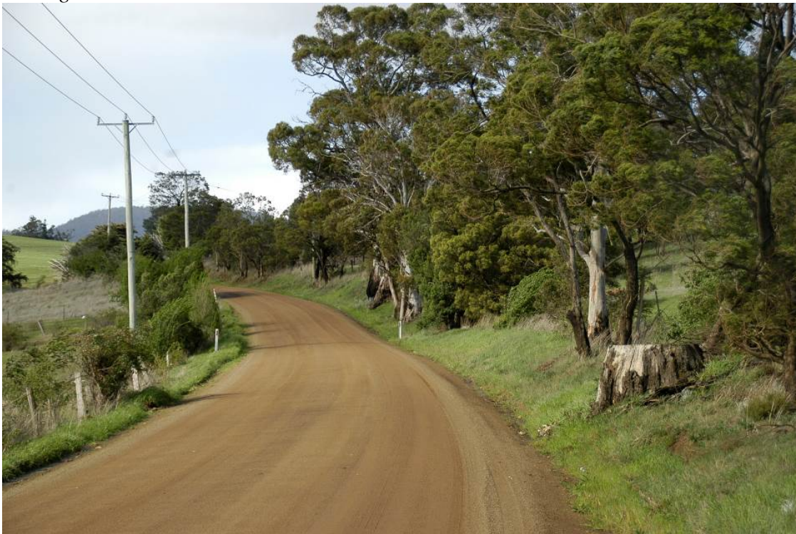
Photo 3_More possible tree removal and embanking may be necessary along this part of the road to achieve a minimum 6m width with shoulders. Photo was taken looking east.
