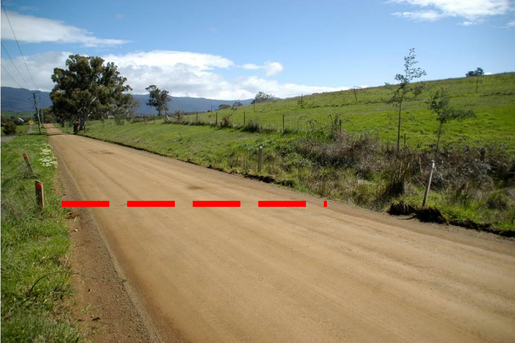
Photo 4_ This culvert would need to be widened to achieve a 6m pavement width with shoulders. The dashed red line marks the approximate position of the culvert. Photo was taken looking west
