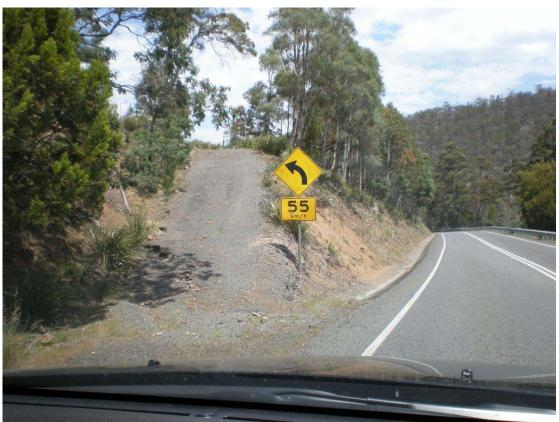
Example of an unacceptable 'access'. This one would give access to Lot 4. Traffic can only enter if travelling south (down the hill) and could only leave by heading north (up the hill). For anybody that wanted to access this lot using this access they would need to find a safe place to turn around and continue on their journey. Note the poor site distance.
