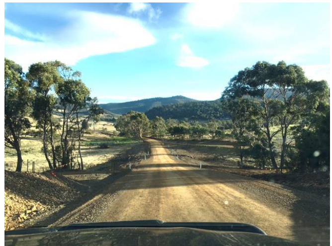
Looking West along Yarlington Road (completed works)
