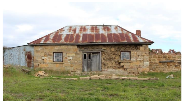
Oatlands Commissariat Restoration Project
