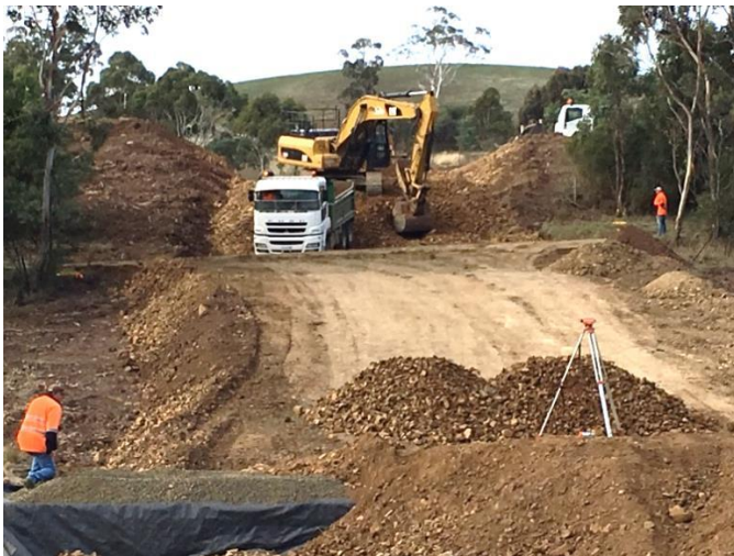
Looking East along Yarlington Road (during construction)
