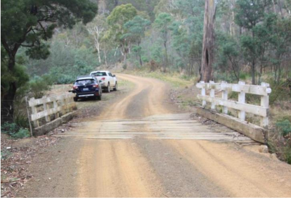
Grahams Creek Road Bridge (existing structure)
