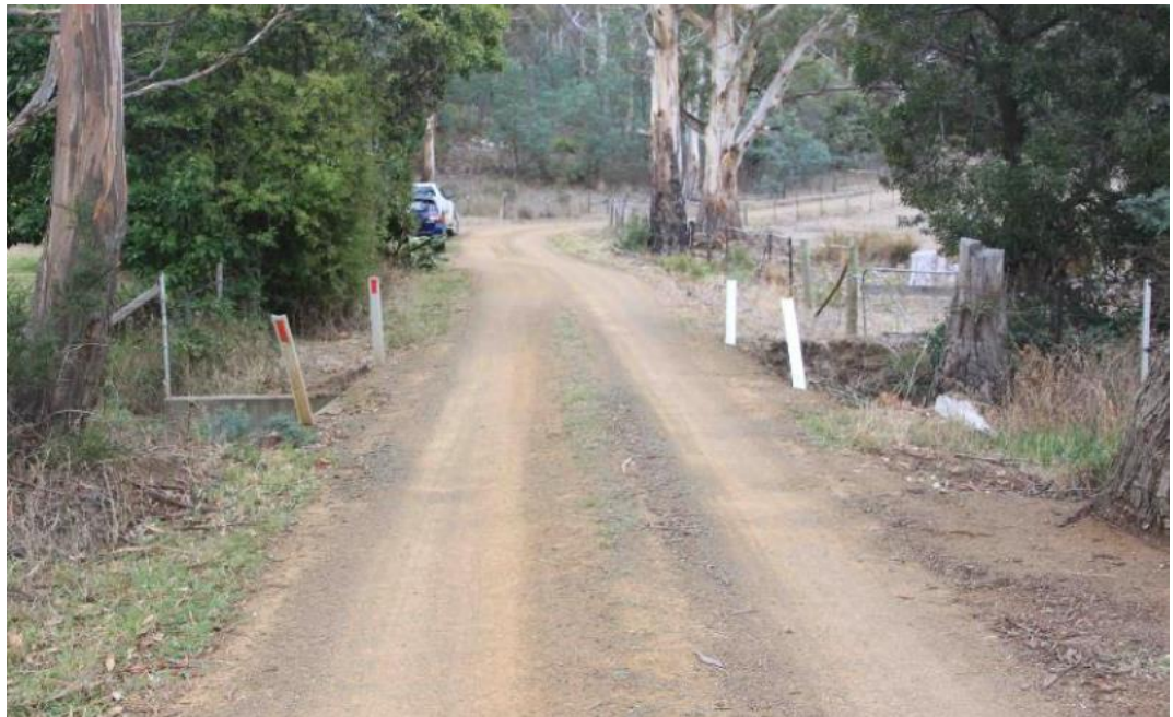
Noyes Road Bridge (existing structure)
