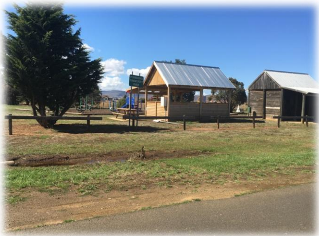
The new BBQ hut at Tunbridge was a request from the local Community to add value to their local park and to cater for travellers along the Midland Highway.
