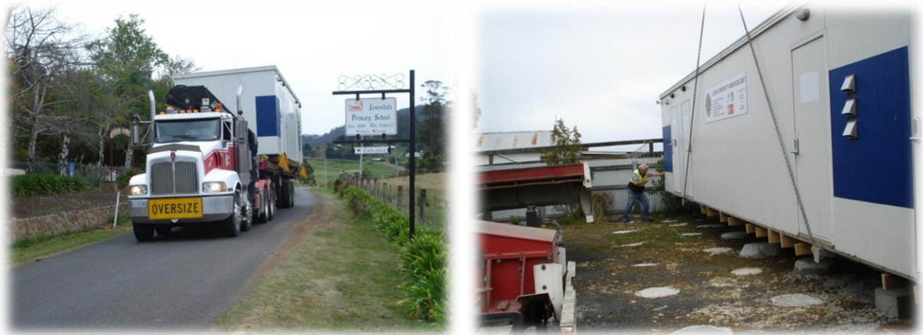
The Lion’s Amenities Facility being transported from Dunalley to Levendale to provide efficient on-site amenities for the Levendale Centre
