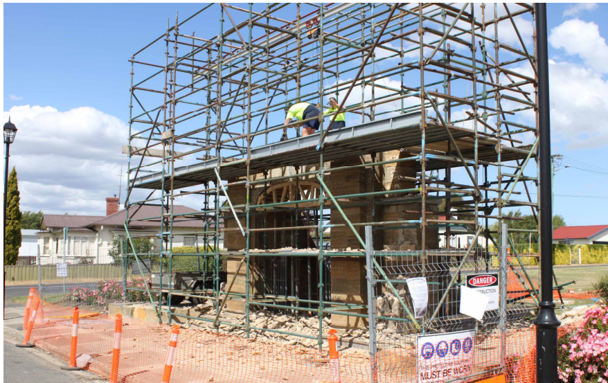
Dismantling and re-erecting the Oatlands Gaol Arch.
