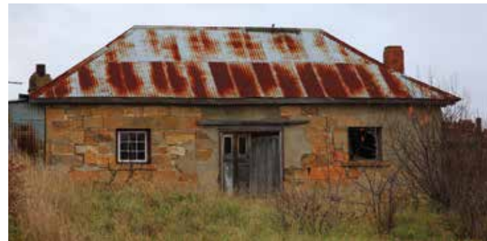
Commissariat's Store and Guard House, 79 High Street
