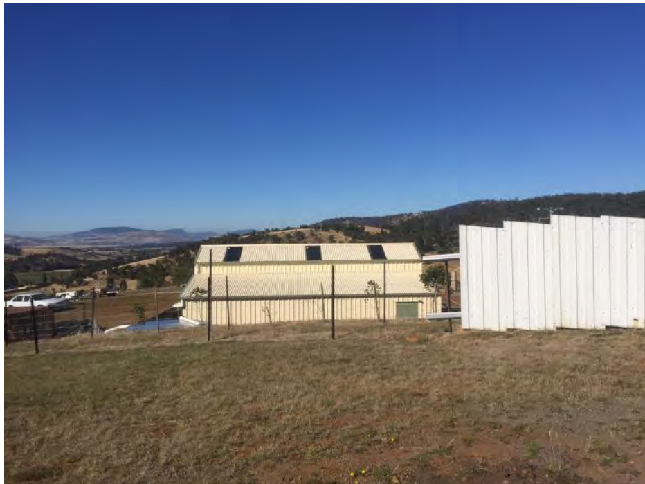
Figure 2. The outbuilding, as viewed from the adjoining property, looking south. The Colorbond fence that has been erected to screen the outbuilding is in the right of the photograph.
