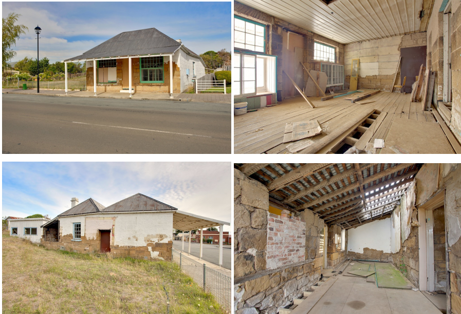
The shop and cottage in front of the commissariat – showing advanced state of decay (photos A. Bewley)
