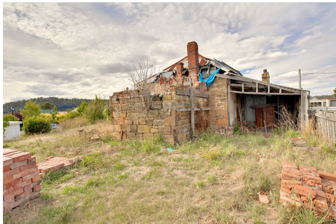
Southern wall of the commissariat (Photo A. Bewley).
