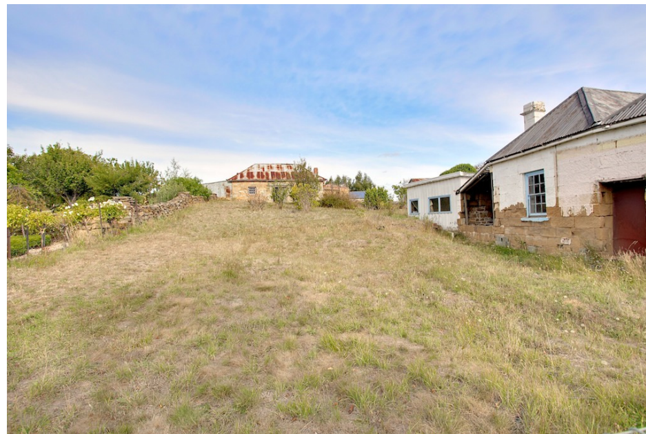
Sweeping frontage to the commissariat from High Street (Photo – A. Bewley).
