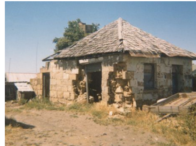
The guard house c1974 just prior to demolition.
