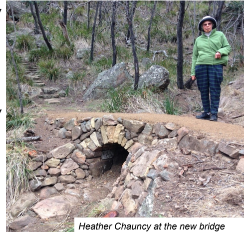
Heather Chauncy at the new bridge
