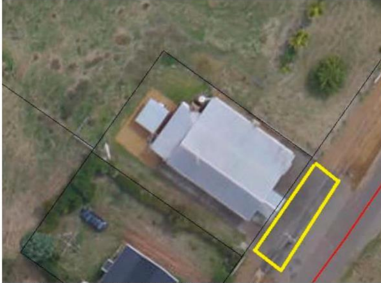
Area 16: Tunbridge Hall; 99 Main Road, Tunbridge
