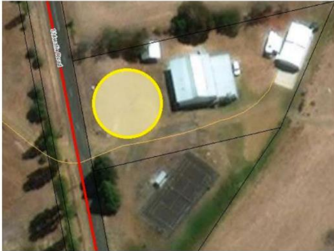
Area 3: Broadmarsh Hall – Car park, 1218 Broadmarsh Road, Broadmarsh
