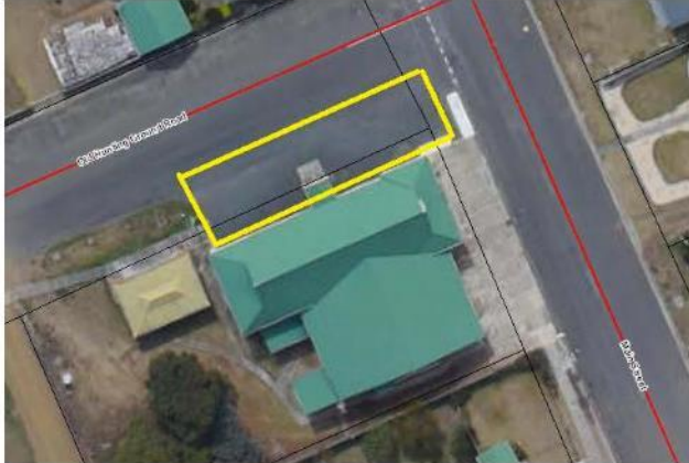
Area 9: Victoria Hall – Old Hunting Ground Road Car Park; 89 Main Street, Kempton
