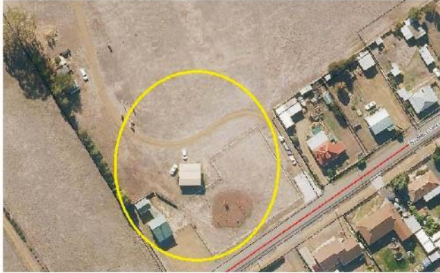
Area 10: Mangalore Oval; 22 Blackbrush Road, Mangalore
