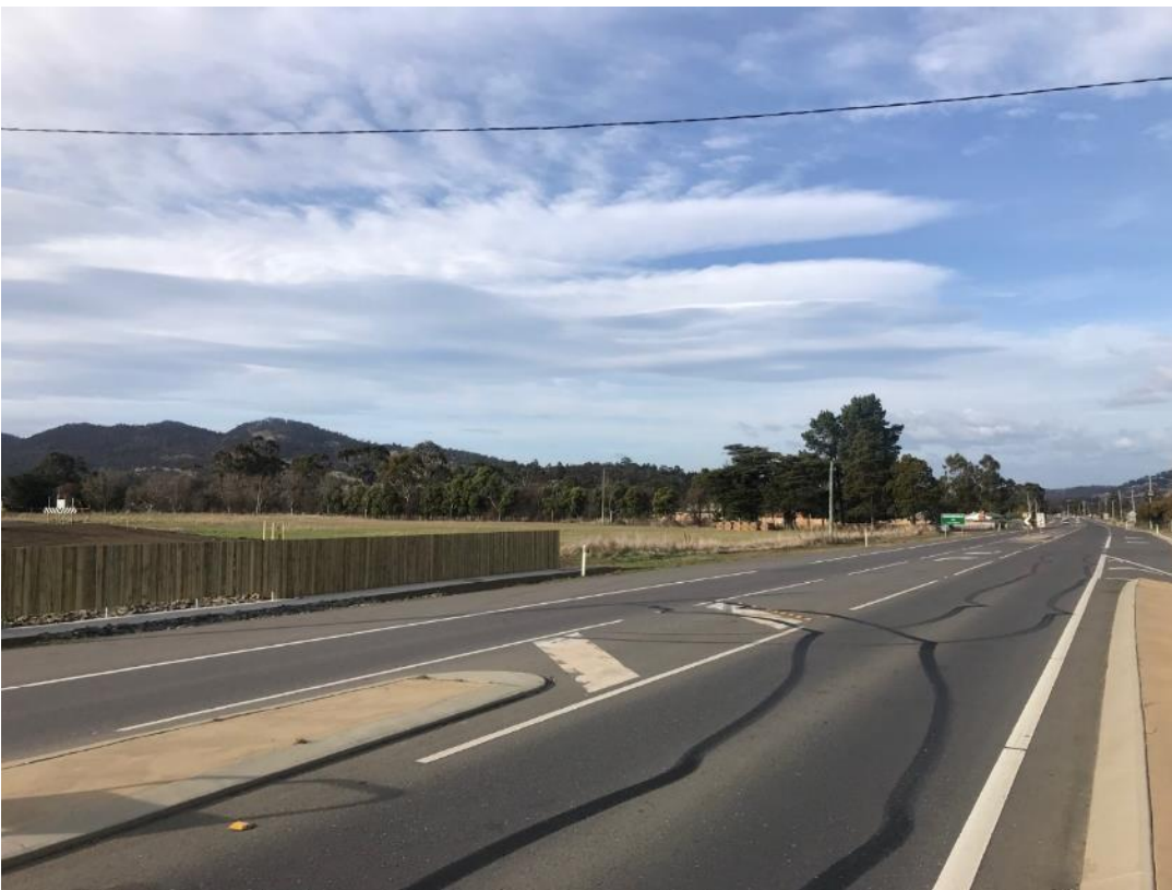
Figure 8: 1844 Midland Highway, Bagdad in streetscape setting (Source: David Cundall, 13 th July 2023)
