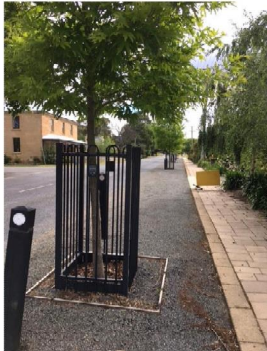
Typical Planting and Surround Tree centre approx. 1m from face of kerb
