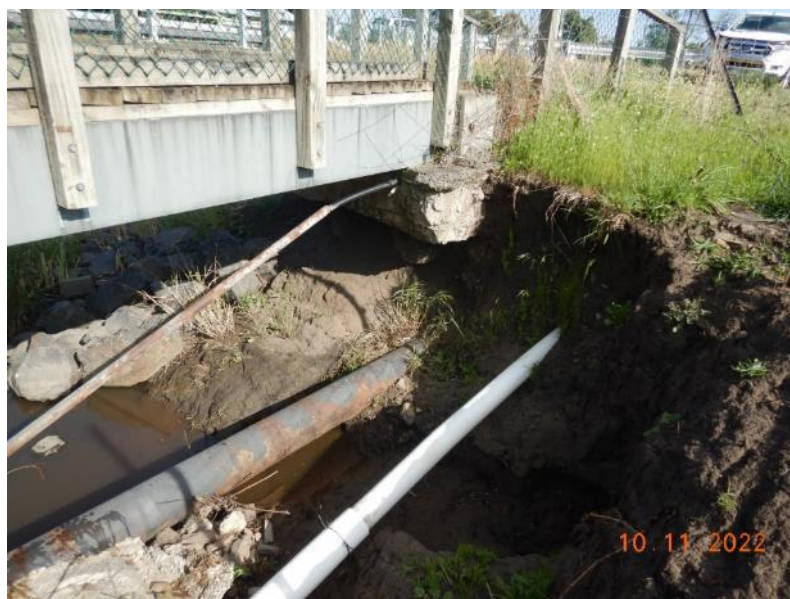
Gangells Lane Footbridge
