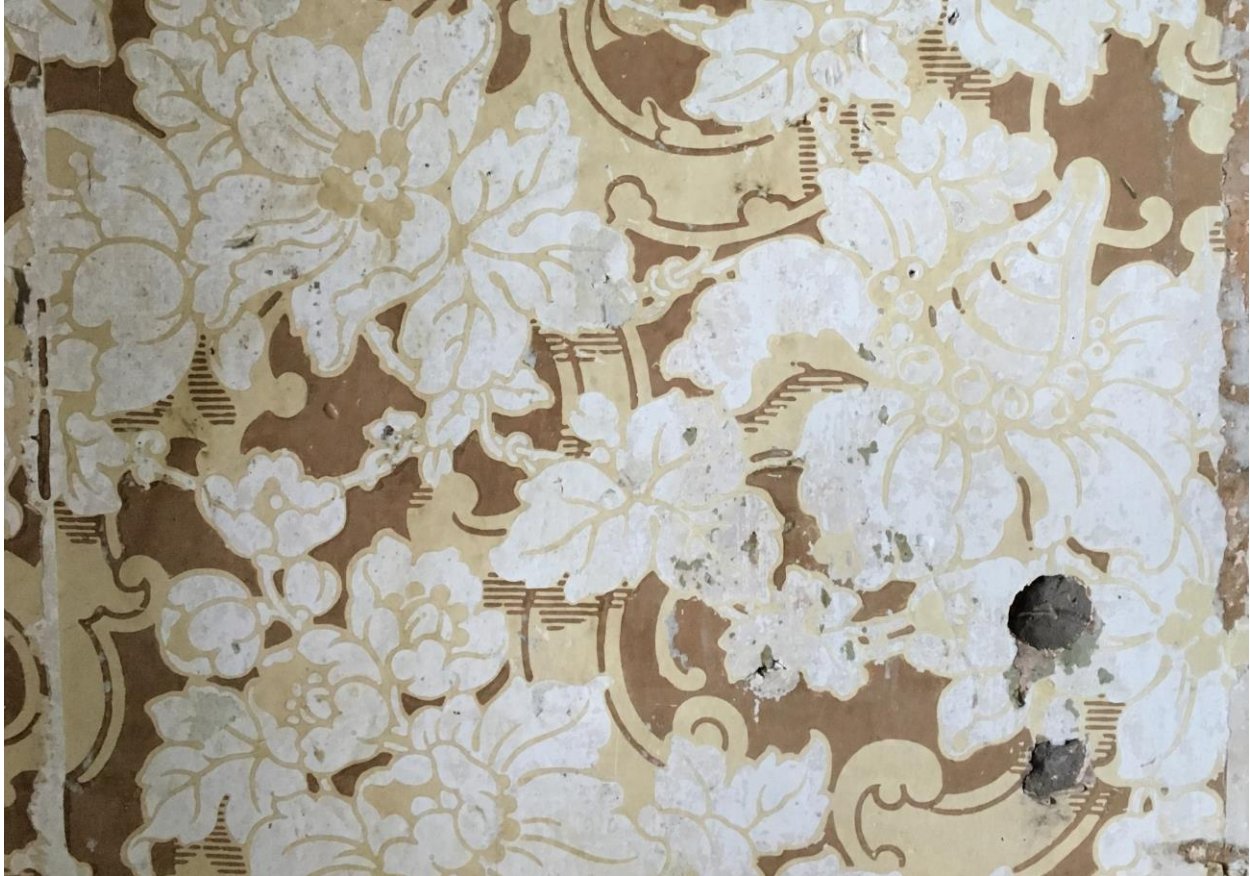
Figure 1: Satin-ground French wallpaper ca 1841, Judge's Chamber (detail). Before being damaged by woodsmoke, UV light and 17 subsequent layers, the white component of this paper (the flowers and foliage) would have sparkled and reflected light as if back-lit. This was achieved by applying multiple layers of the 'ground' colour and then polishing it with French chalk and steel rollers to provide a glossy, reflective surface. The brown and cream layers were then woodblock printed onto the white, giving the illusion that the background colour is the foreground.
