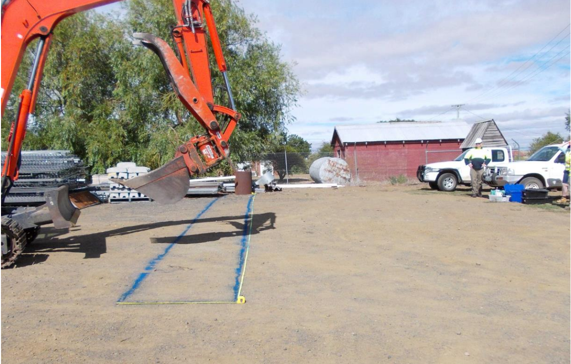
Figure 4.2 – Pre-excavation overview of the trench location (facing south).
