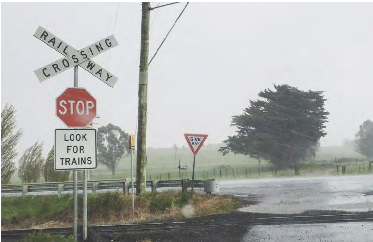
Figure 3.2 : Glen Morey Road Level Crossing
