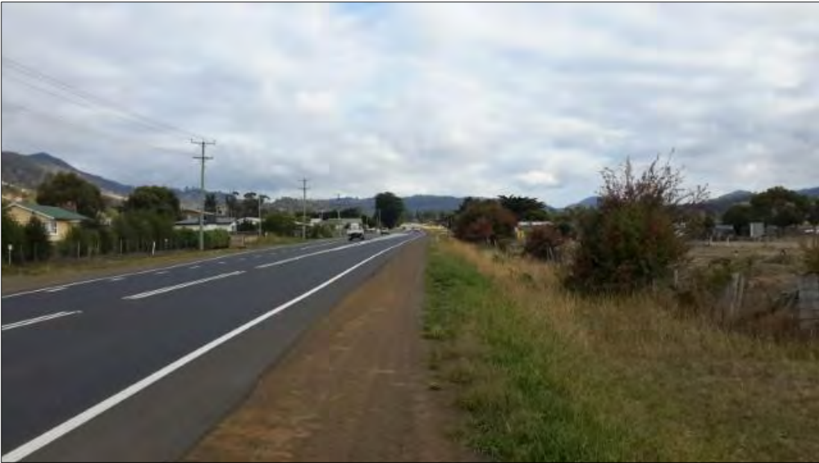
FIGURE 10: SOUTH OF BLACK BRUSH ROAD LOOKING NORTH
