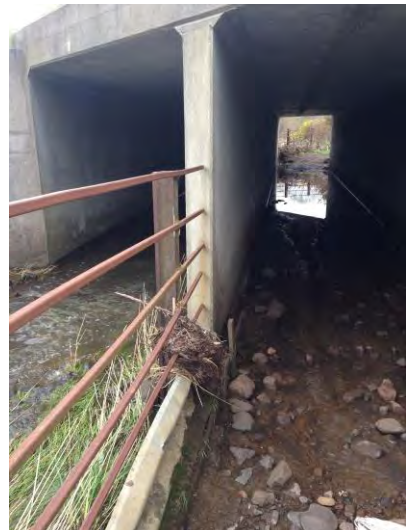
Currajong Creek Culvert
