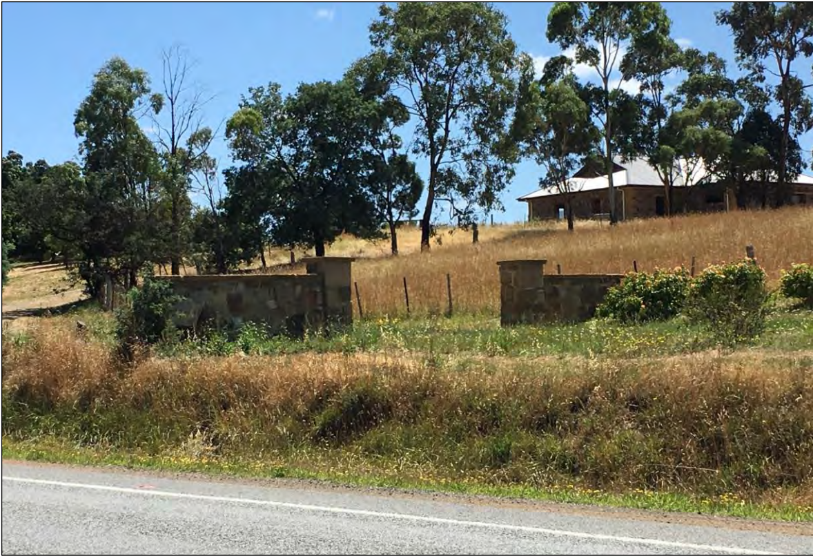
FIGURE 8: RECENTLY CONSTRUCTED ENTRY FEATURE TO CORNELIAN HILL
