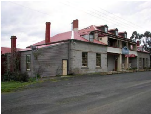
Figure 39 - Hamilton Hotel, Tarleton Street
