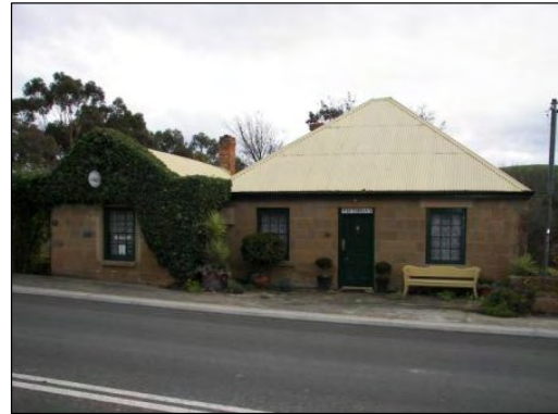
Figure 40 - George and Victoria's Cottages, Franklin Place, Hamilton
