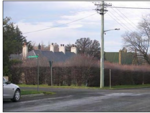
Figure 62 - The Chimneys (former convent), Richmond Street
