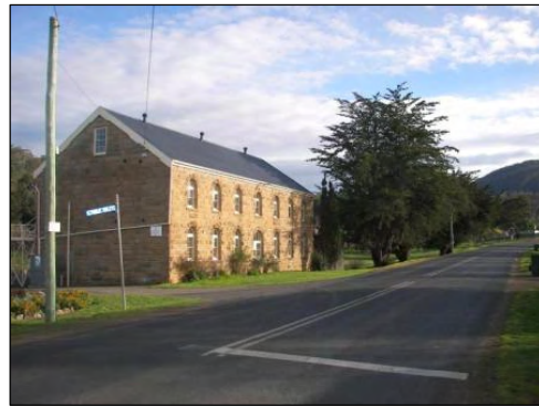
Figure 56 - Campania Mill, Reeve Street
