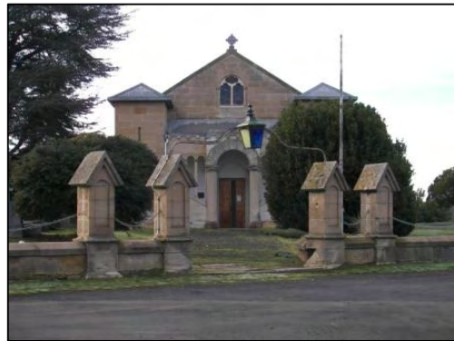
Figure 25 - St Marks Church, Pontville
