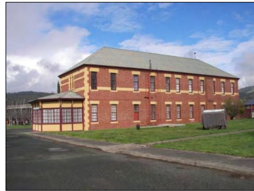
Figure 43 - Masonic Lodge (former Female Ward K2)
