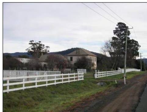
Figure 68 - Woodburn House, Midland Highway
