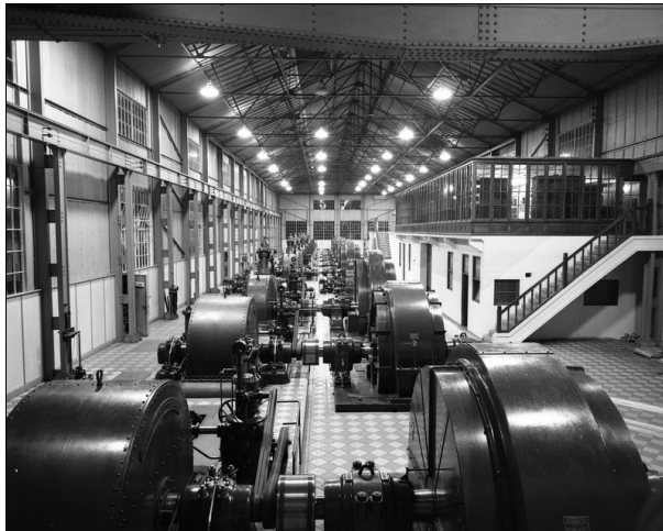
Figure 8 - Interior Waddamana Power Station (c.1950s)
