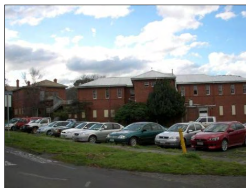
Figure 45 - Esperence House, Willow Court
