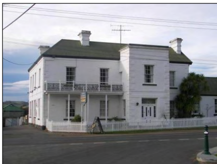
Figure 57 - Former shop, Reeve Street
