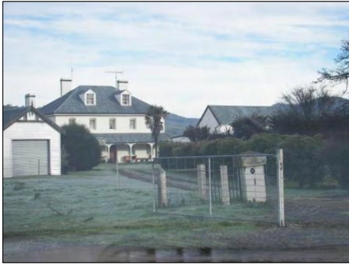
Figure 65 - Oakmore homestead and outbuildings
