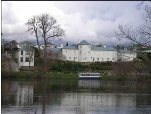
Figure 50 - Woodbridge House, Bridge Street
