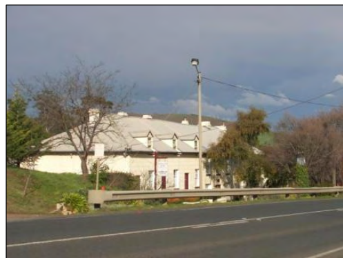
Figure 29 - The Barracks (Lythgo's Store)
