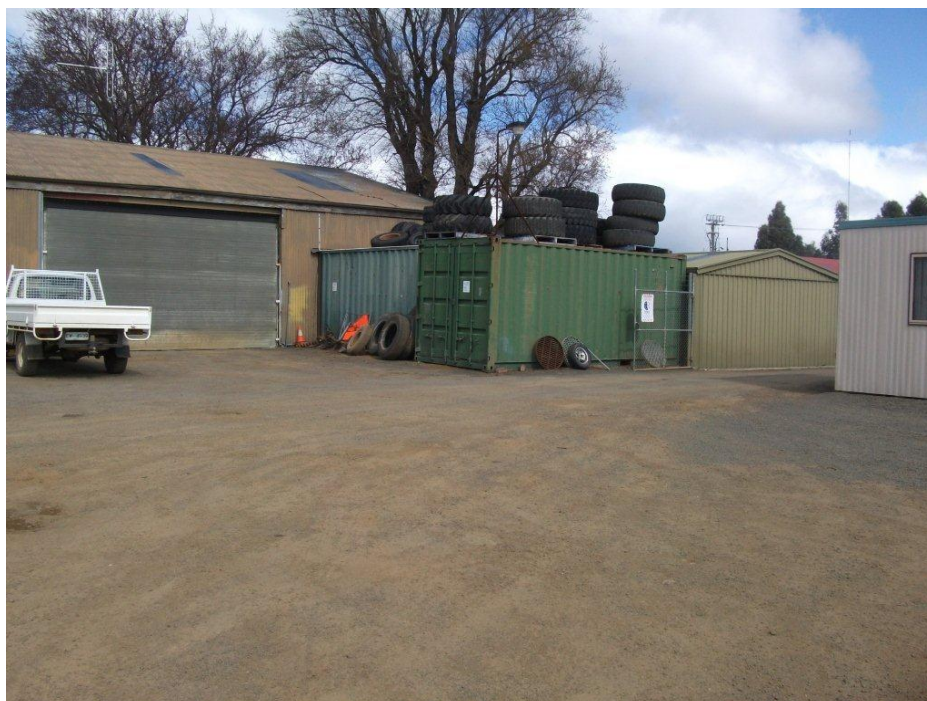
Plate 5: Site of UST 1 (decommissioned)
