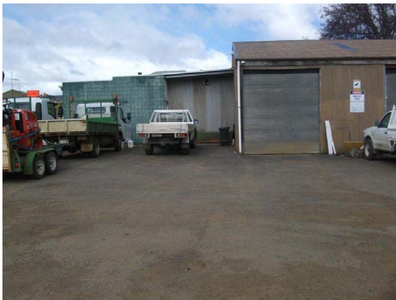
Plate 8: Location of Original Oil Store
