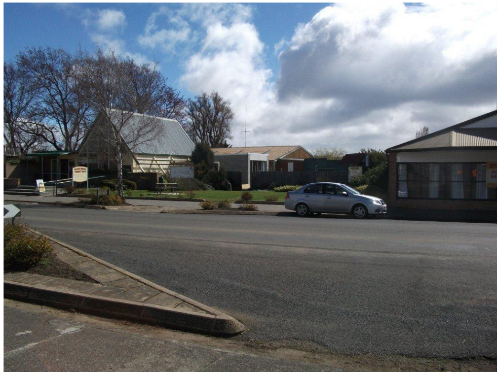
Plate 1: Site Viewed from High St.
