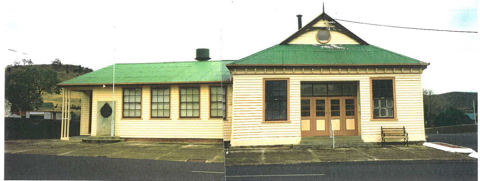
MEMORIAL HALL Form a pleasant pedestrian area in front of formal entry doors Toilet block visually clashes with the hall.
