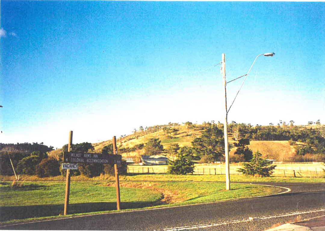
Sign not straight and not well placed. Lighting insufficient light pole inappropriate.
