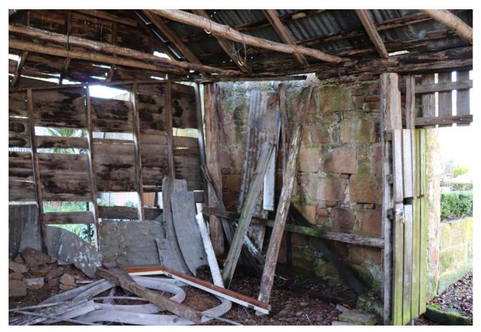
Failed wall framing, lack of base plates and discharge of rainwater onto significant stone wall (to be retained).
