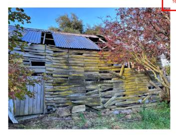
The back exterior of the shed is completely weather worn, rotten and the roof sheets are completely unsafe.
