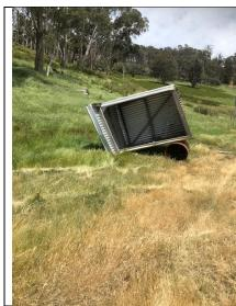
The shelter at the gate needs to be up righted and fixed. Requires slab to AS2870 and fixing/ bracing to be in accordance with AS1684
