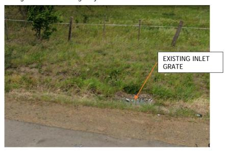
Image 7 - Existing Inlet Pit Midland Highway Table Drain
