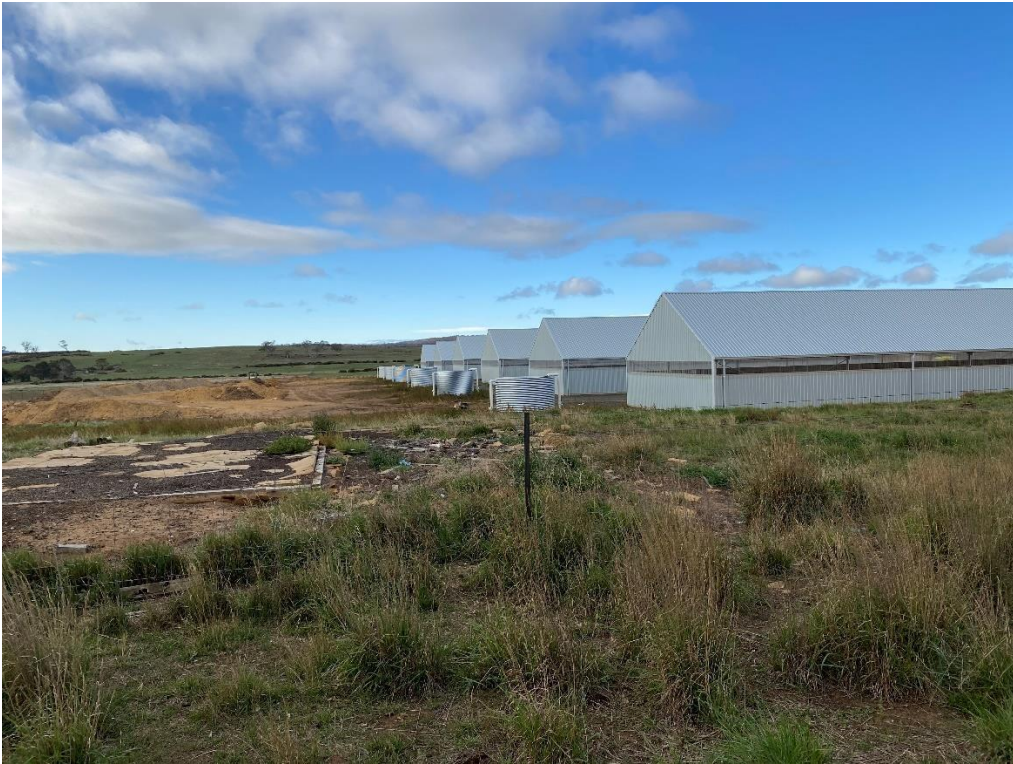
Photograph 5: View from Hastings Street road reserve of rear of existing Bond Stores with water tanks
