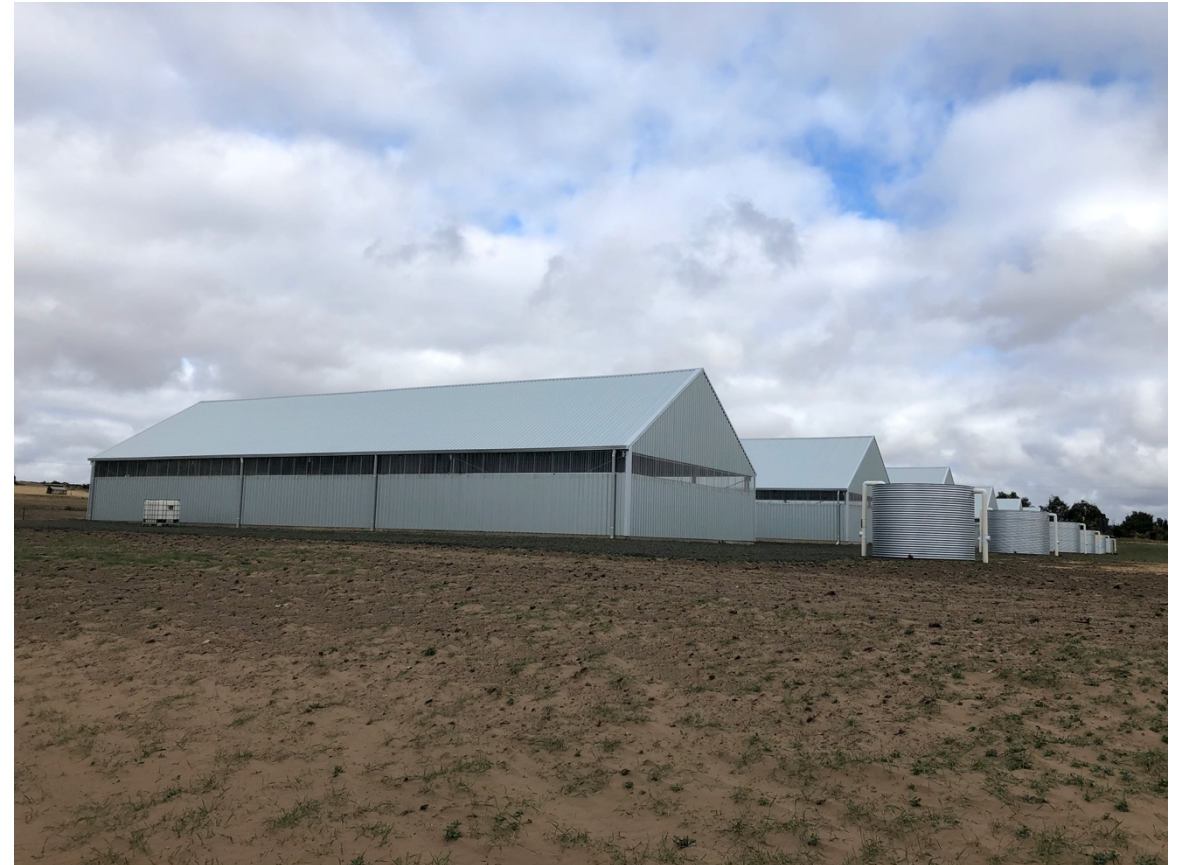
Existing sheds: view from Bentwick Street boundary, showing ends (and water tanks) facing Tunnack Road. Proposed sheds to be located to the right.
