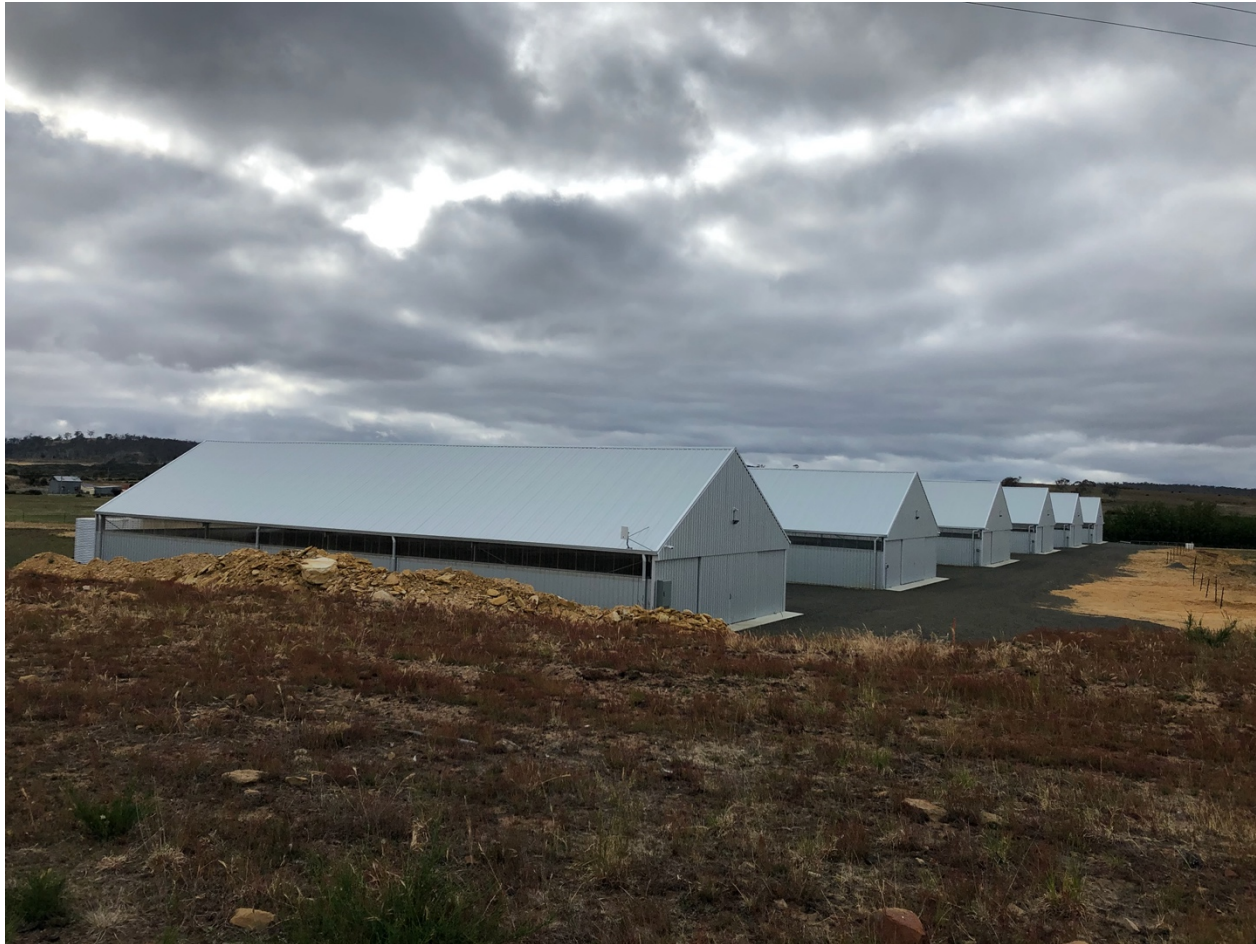
Existing sheds: view from Hastings Street boundary showing rear walls (facing away from Tunnack Rd)
