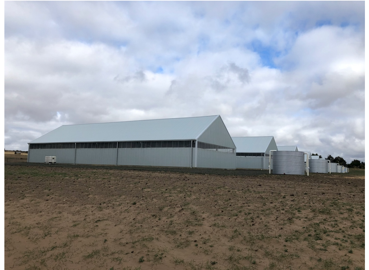
Existing sheds: view from Bentwick Street boundary, showing ends (and water tanks) facing Tunnack Road. Proposed sheds to be located to the right.
