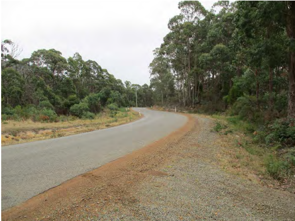
Photograph 6.5: View to north along Woodsdale Road from the northern driveway
