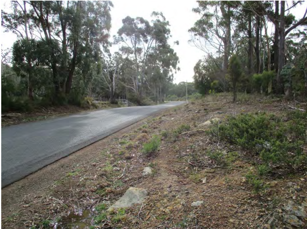
Photograph 6.1: View to north along Woodsdale Road from the southern driveway
