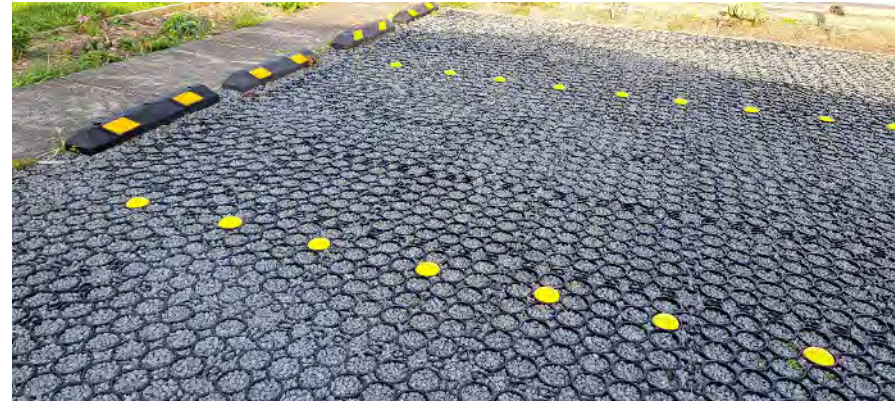
Figure 7 Image of Tru grid pavers installed in Kingston driveway.
