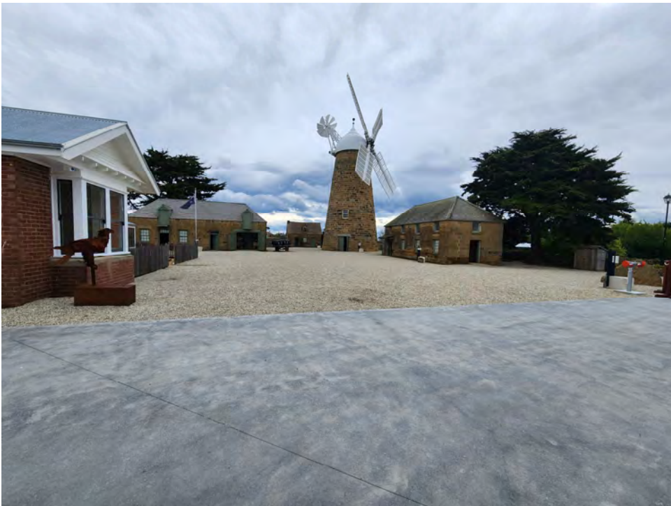
Heritage buildings and adjacent new concrete pavement. Photo by Hamid Saeidi
