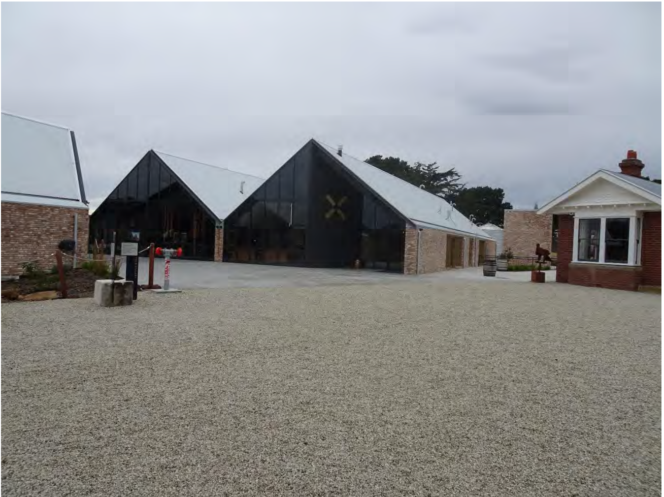
Image.5. New distillery buildings at 99 High Street in the centre and left of the image which are located internally within the subject site. The adjacent red brick miller's Cottage can be seen on the right. Gravelled landscaping in the foreground is located within the Callington Mill site at 6 Mill Lane.
