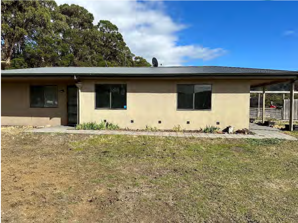
Figure 8 - Existing dwelling and managed land within Lot 1, view facing W
