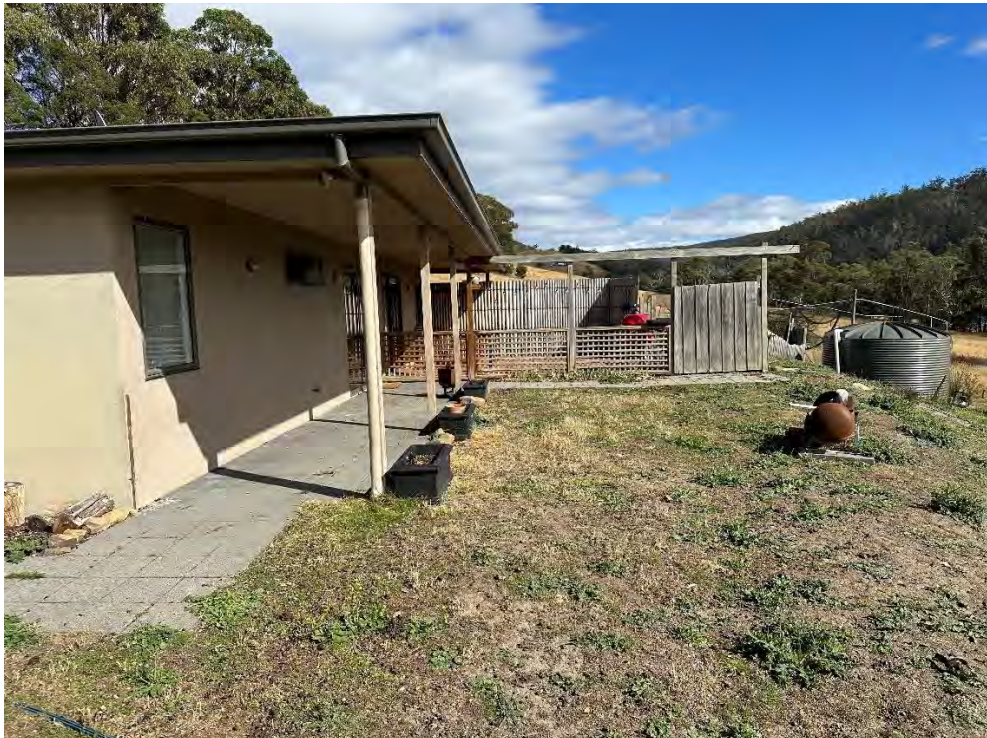
Figure 9 – Existing dwelling and managed land within Lot 1, view facing W
