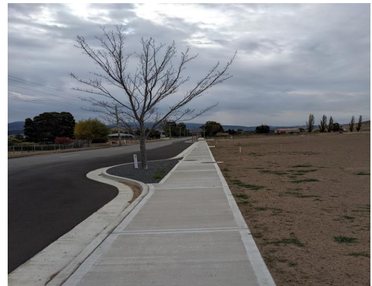
Footpath, Main Street, Kempton
