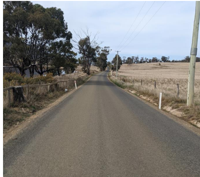
Re-Construction of Native Corners Road
