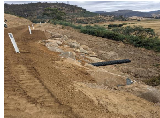
Landslip Repair Clifton Vale Road
