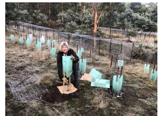
Revegetation work at Chauncy Vale
