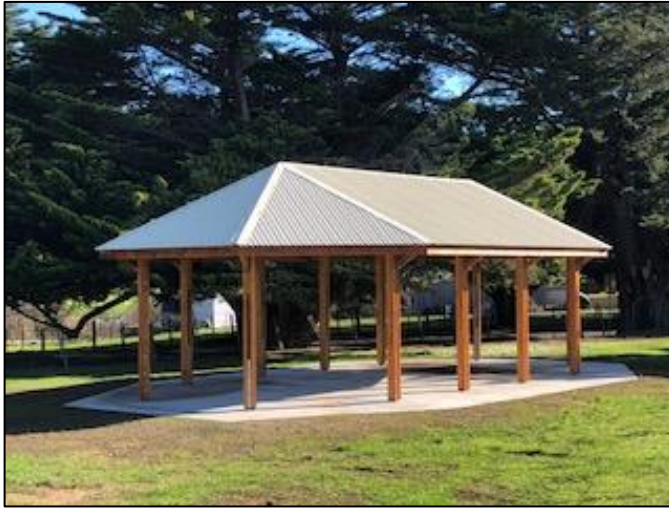
Memorial Avenue Shelter – Kempton
