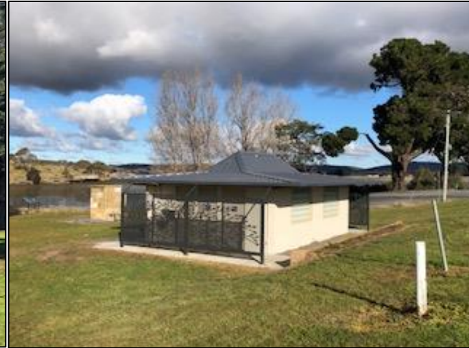
Refurbishment of the Oatlands Toilets at the Esplanade
