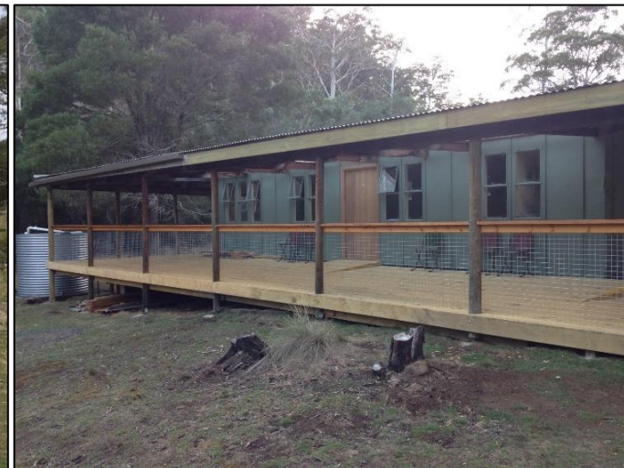
Chauncy Vale building refurbishment
