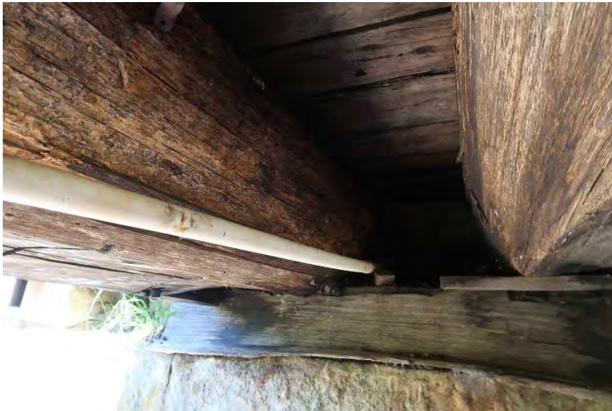
Figure 6: Timber girders and spreader at southern abutment
