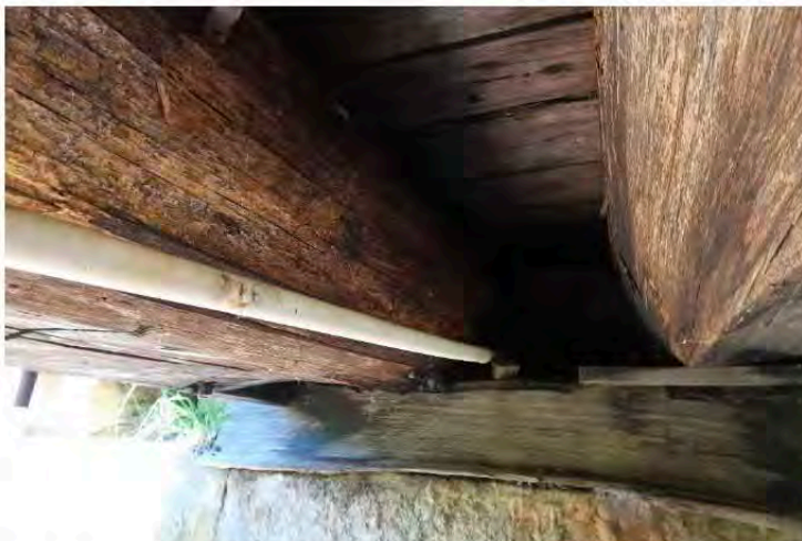
Figure 6: Timber girders and spreader at southern abutment
