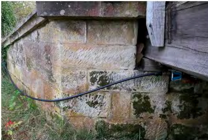
Figure 9: Face of northern abutment
