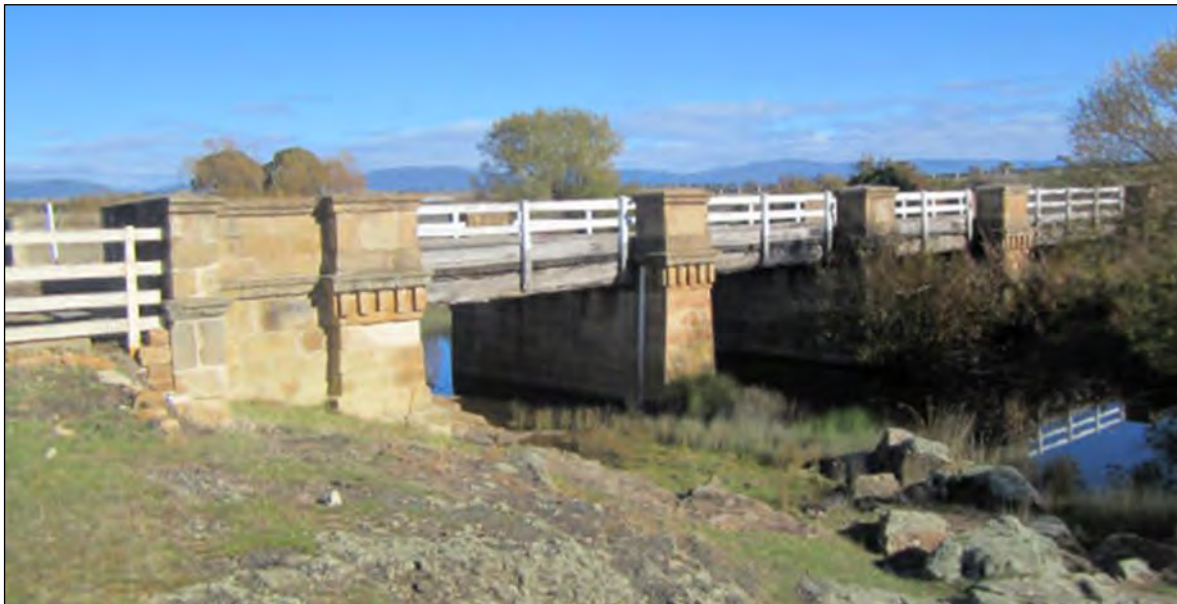
PLATE 1 VIEW OF THE BRIDGE FROM UPSTREAM (EASTERN BANK)
