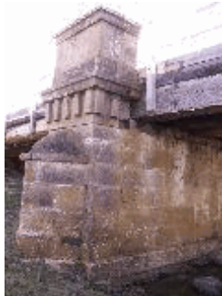
Tunbridge Bridge pier
