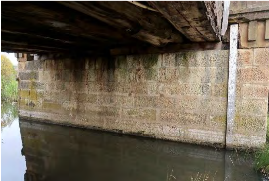
Figure 8: Southern face of the southern pier 1
