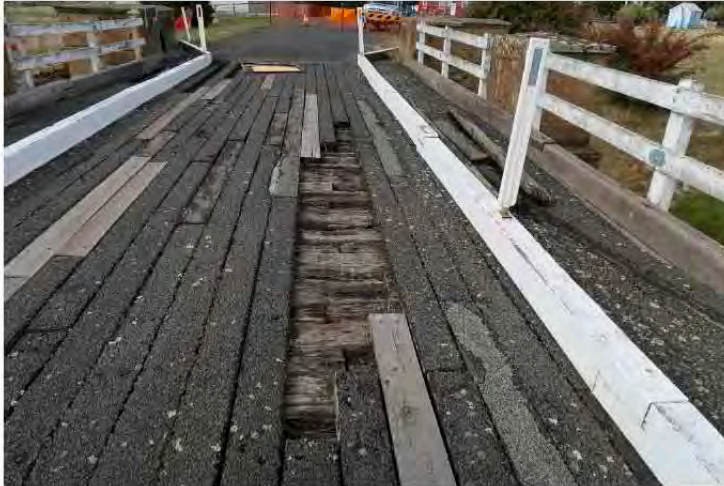
Figure 7: Deck condition
