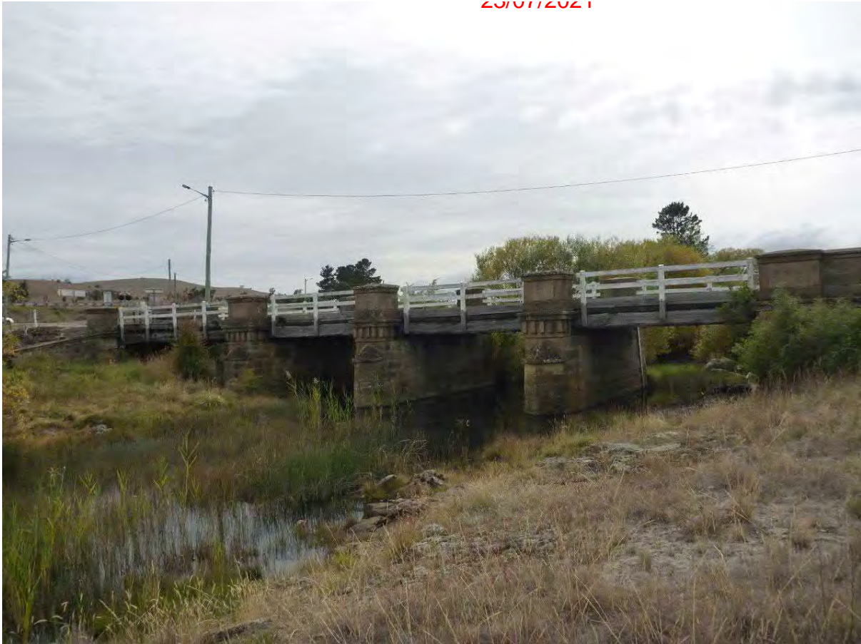
Figure 2: The Blackman River Bridge view of the upstream facade, looking to the north east (2015).
