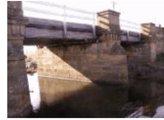
Timber deck and stone pier
