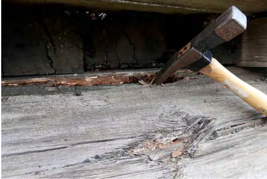
Figure 5: Condition of girder - northern span, western external girder
