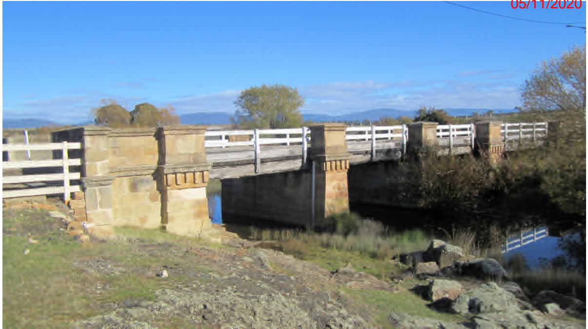
Photograph 1. NE downstream face of bridge.
