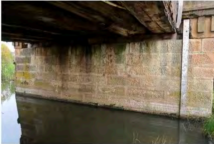
Figure 8: Southern face of the southern pier 1
