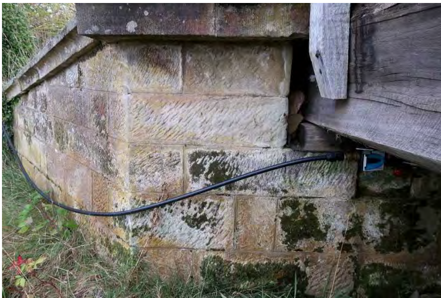
Figure 9: Face of northern abutment
