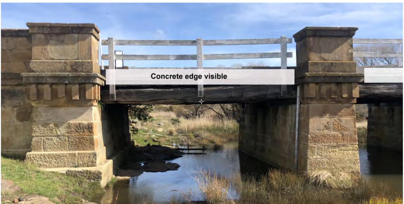
Approximate area of visible concrete edge that would arise from this proposal.
