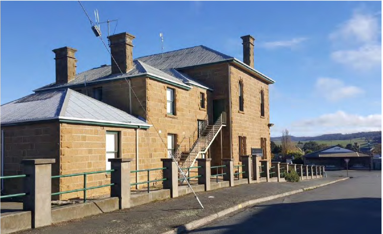
Image: Old Council Chambers – Building step up in scale. Roofs tucking un under other roofs, stone cladding, steel roofs PLA image
