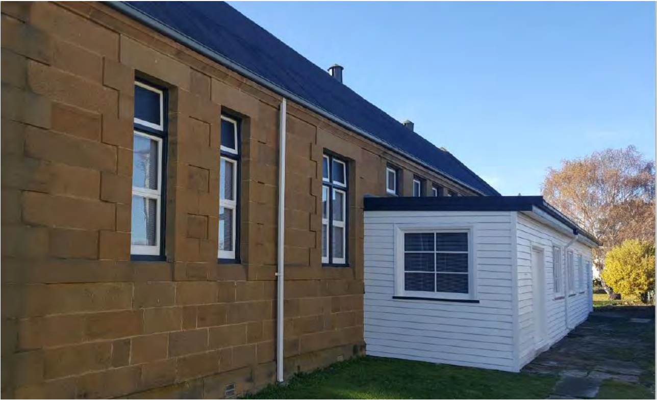
Image: Old Oatlands Courthouse – mix of roof forms and pitches. Awning skillion roof to the side of the building, and a mix of cladding materials – sandstone and timber weatherboards PLA image
