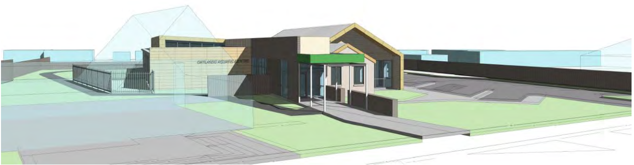
Image: Oatlands Aquatic Centre – image of the proposed new facility looking North from High Street
