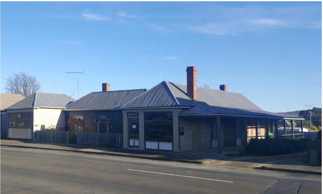
Image: High Street streetscape – mix of roof forms and windows.
