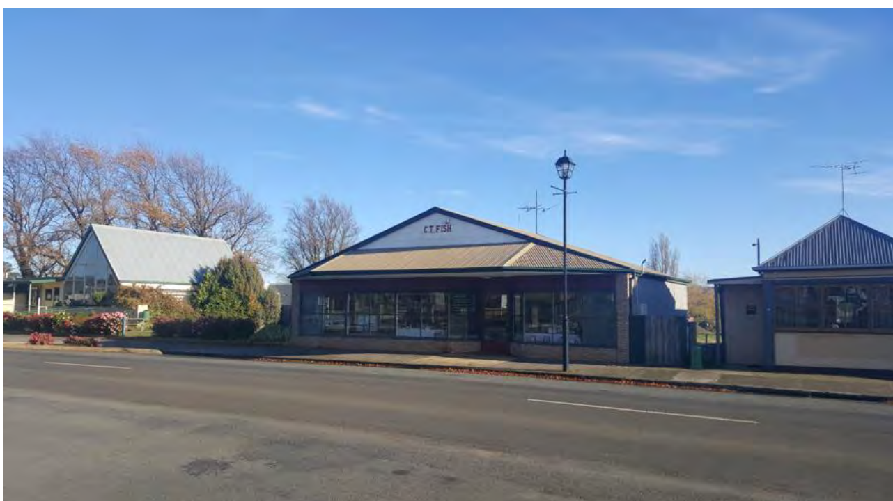
Image: Site from High Street looking West – CT Fish building foreground (to be demolished)
