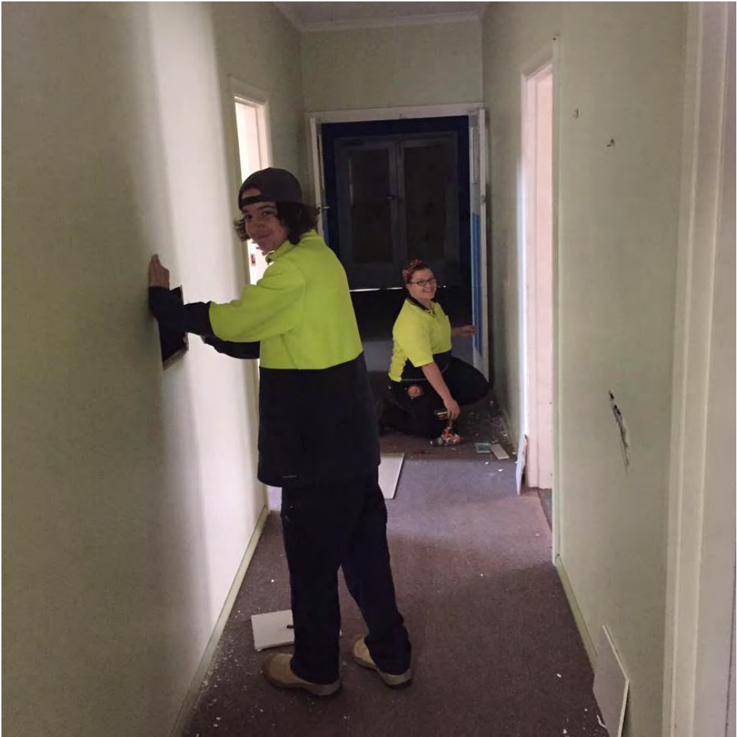
Plaster repairs in progress
