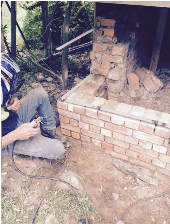
Repairing brickwork on the veranda plinth
