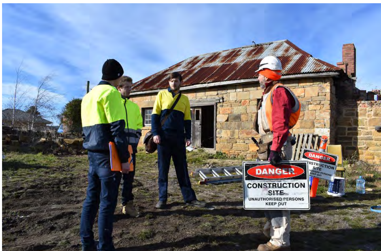
Trainees first-day on site receiving inductions
