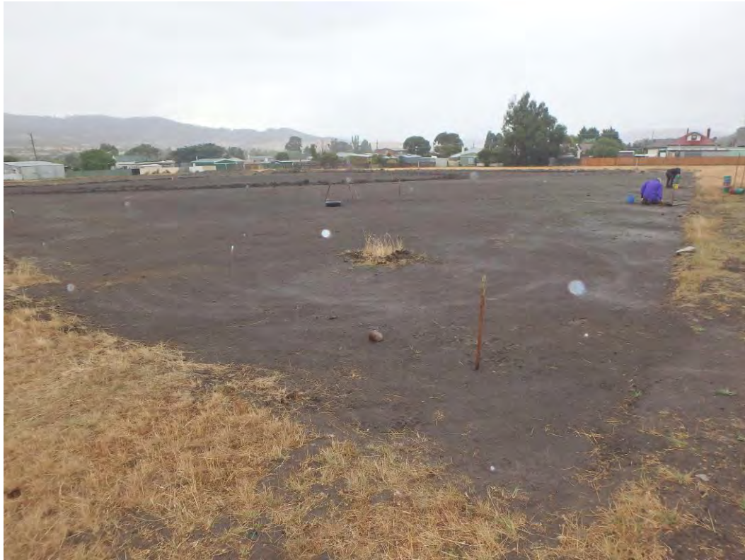
Plate 1: View south-east across the west portion of the horse arenas footprint, where the 15 test pits were placed
