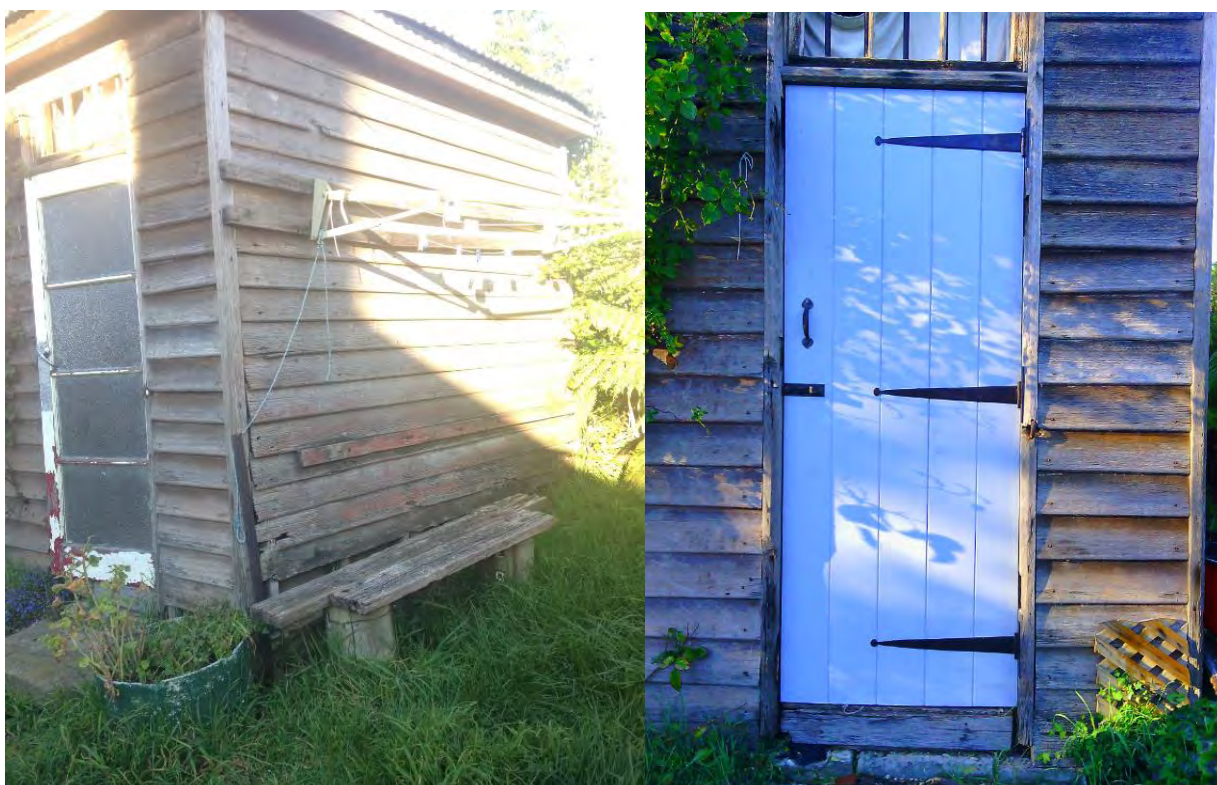
Repairs to cell block joinery, cladding and door
