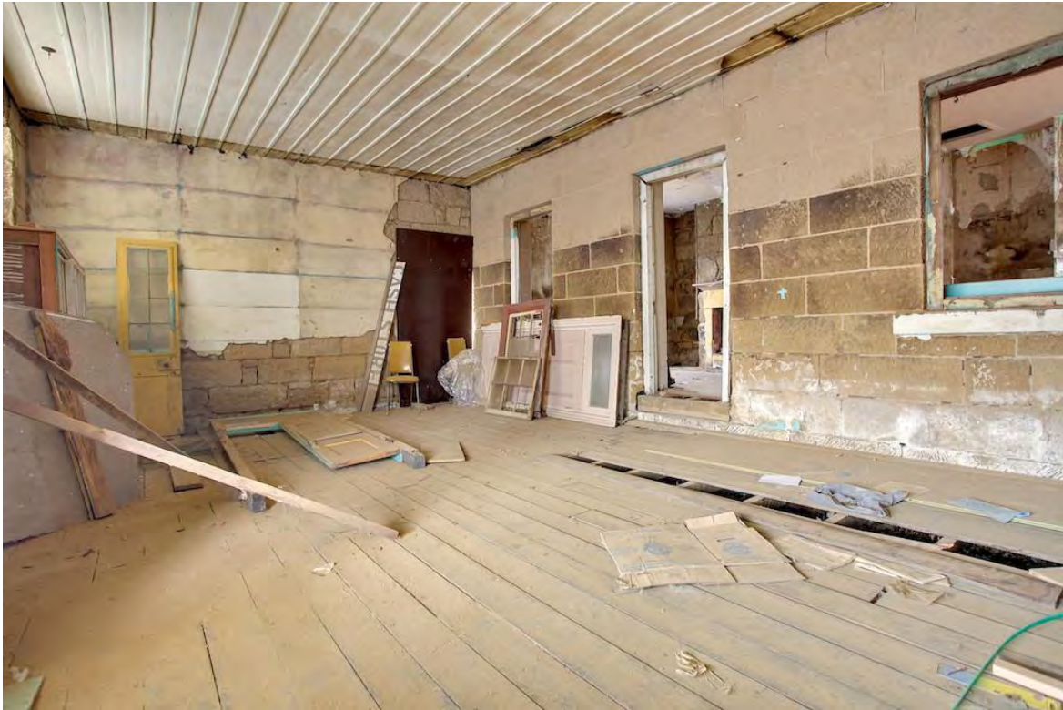
Before – participants worked on the new floor and surface finishes.
