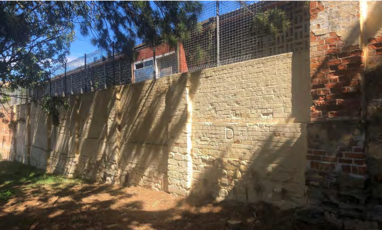
Willow Court walls - after
