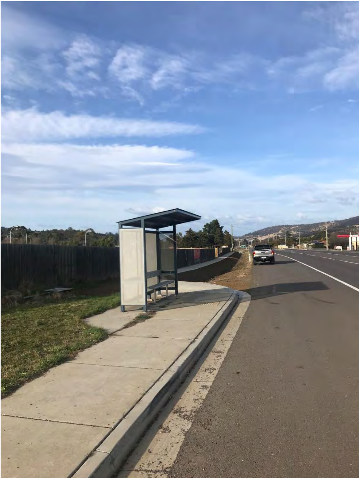
Figure 4: Photo of bus stop on eastern side of Midland Highway with footpath towards 1844 Midland Highway (Source: David Cundall, 13 th July 2023)
