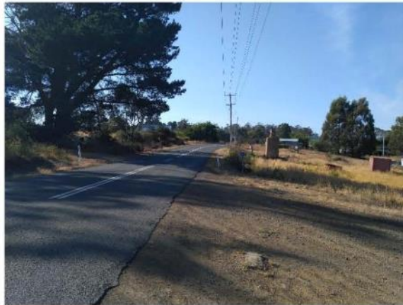
Photo 1 – Tunnack Road looking south from the siding access intersection.
